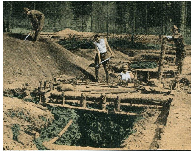
ONE OF THE ARTS OF WAR—TRENCH DIGGING IN CAMP LEWIS
